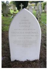
steel dowels. The bottom of the new headstone was drilled to accept the dowels and was further supported by two stone blocks against the front and back as haunching. Only the stone itself remains visible above the ground.
