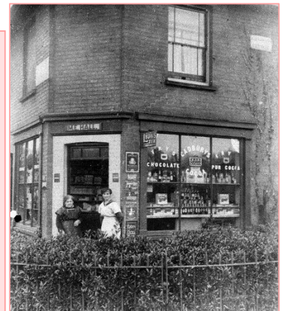
Post Office – Roy Brinton Shop opposite the post office RSHG
